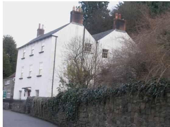
Fig.58 Crown Lodge. The typical double pile (twin roof) of this 18 th century house is apparent from this view. The symmetry of the Georgian façade and the proportions of the windows are characteristic of the period.
