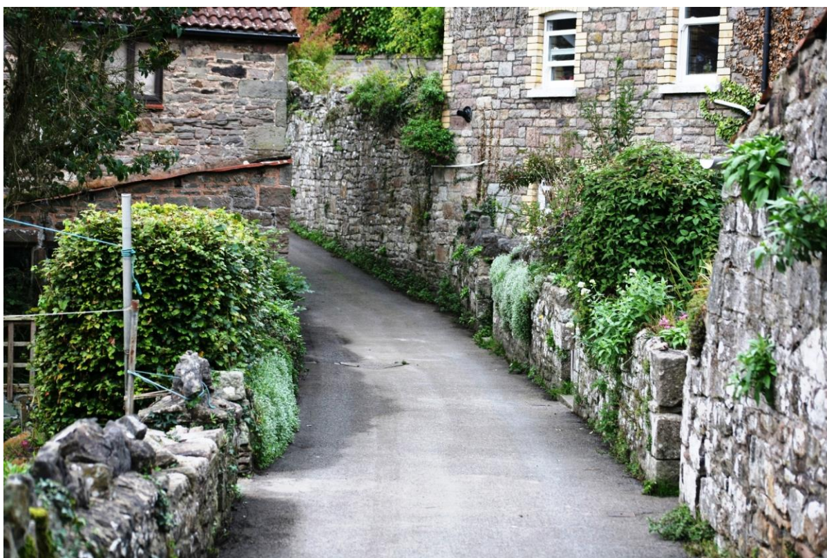
Fig.79 Boundary walls are a key feature of most of the Conservation Area. In this example, walls, retaining walls, boundary walls and the sides of buildings combine to strongly define this narrow lane leading to St Michael's Church.
