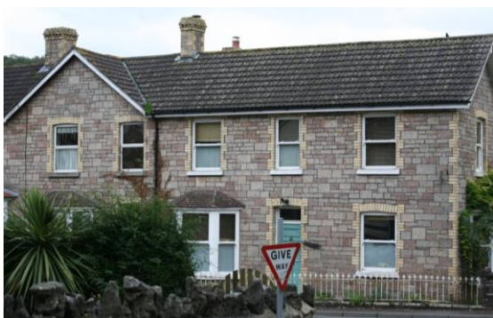
Fig.15 Wyeborne and Redborne; terraced houses
