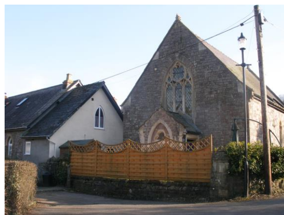
Fig.61 The former non-conformist chapel, now converted to residential use
