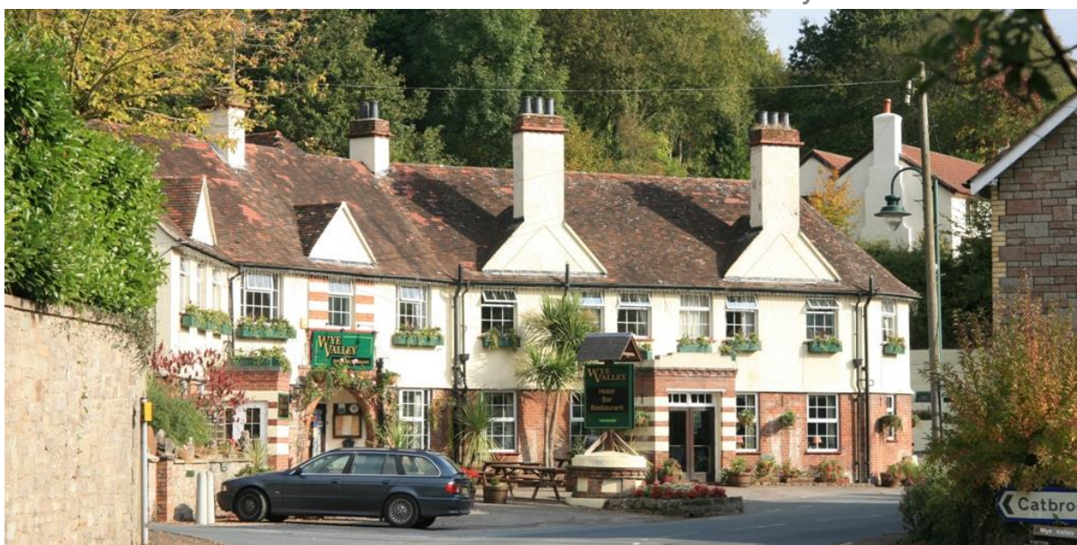
Fig.21 The Wye Valley Hotel (circa 1920) displaying a good and varied mix of materials reflecting the trends of the architectural period
