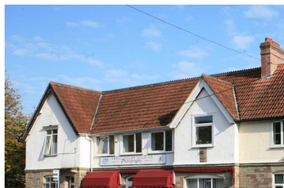
Fig.78 The use of clay pantiles is a key characteristic of some parts of the Conservation Area, particularly the commercial areas to the abbey environs
