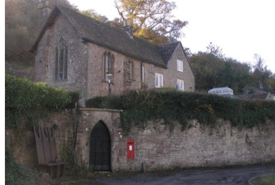
Fig.51 St Anne's House stands above the main road opposite the Abbey. It was originally a chapel associated with the Abbey gatehouse. The medieval portion is on the left and a 19 th century extension to the right.
