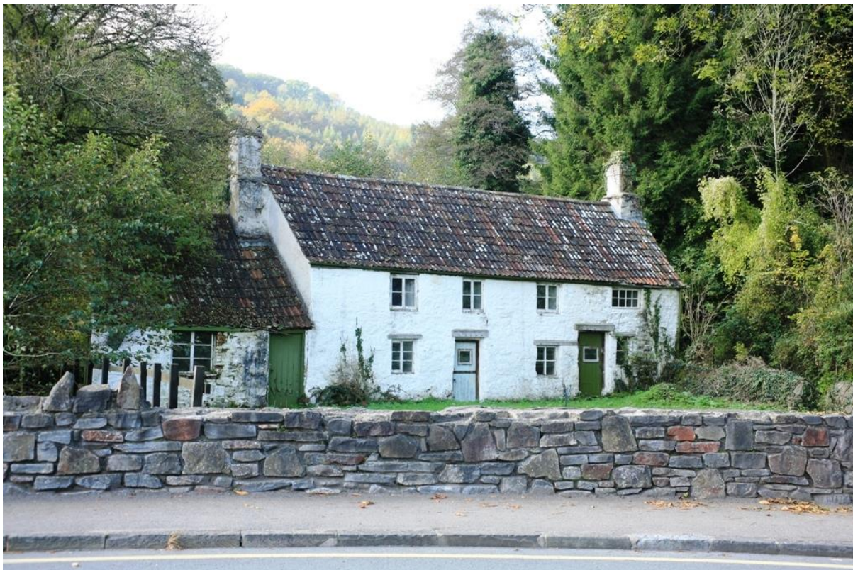
Fig.32 The Bay: attractive and largely unaltered vernacular stone cottage, presently unoccupied and as such a vulnerable heritage asset within the Conservation Area
