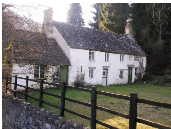
Fig.53 Former cottages north of the Royal George Hotel, now one house known as 'The Bay'. These examples are remarkably free of alterations and retain an authenticity of traditional cottage design
