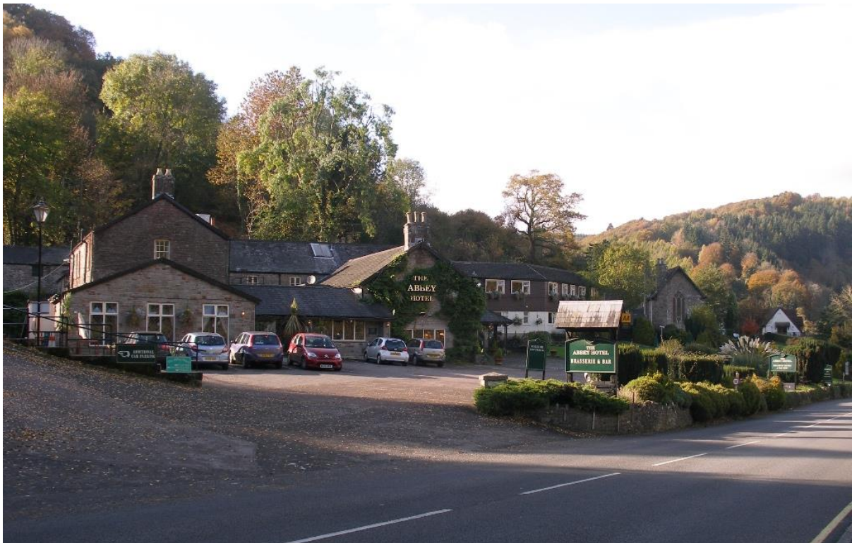
Fig.68 The Abbey Hotel. This low profile extensive composition has a 19 th century core built into the hillside, backing onto a lane to the rear.
