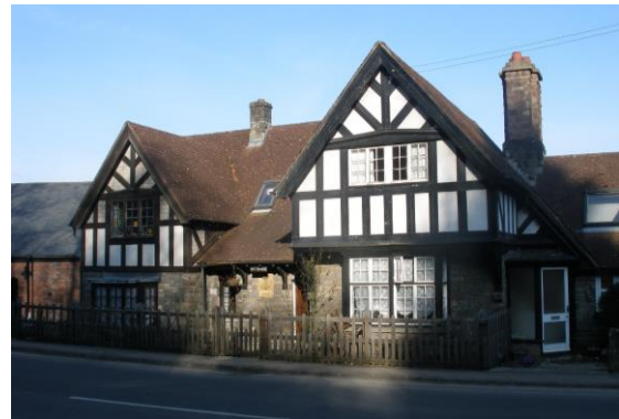
Fig.69 Wye Cottage, built in 1903 in the Domestic Revival style, recalls the medieval hall house type, with its gabled and timber framed cross wings. Both this and a number of cottages in Tintern display the Royal cipher denoting their Crown status.
