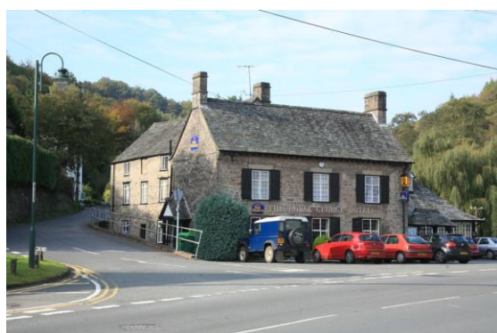
Fig.31 The Royal George: a landmark corner building of historic and architectural interest and forming an important group with Crown Lodge and Walnut Tree Cottage
