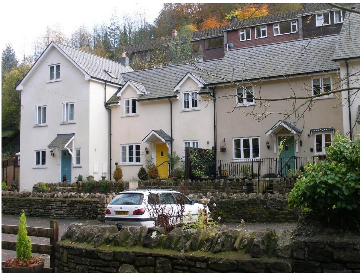
Fig.74 Recent terrace in the Angiddy valley. An unassuming terrace, utilising subtle variations in eaves heights and building alignments to create an informal character.
