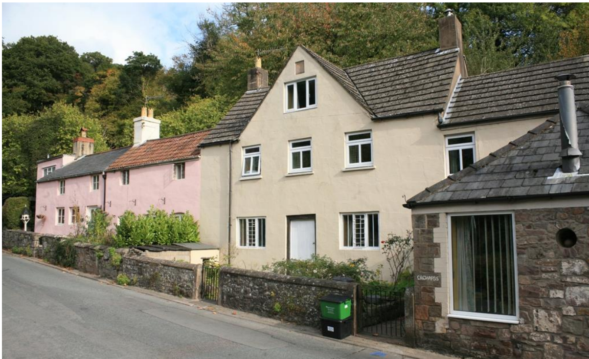
Fig.18 Orchard House, Rocklea & Rose Cottage: An attractive and varied group making a positive contribution to the Conservation Area notwithstanding out of character alterations to windows.
