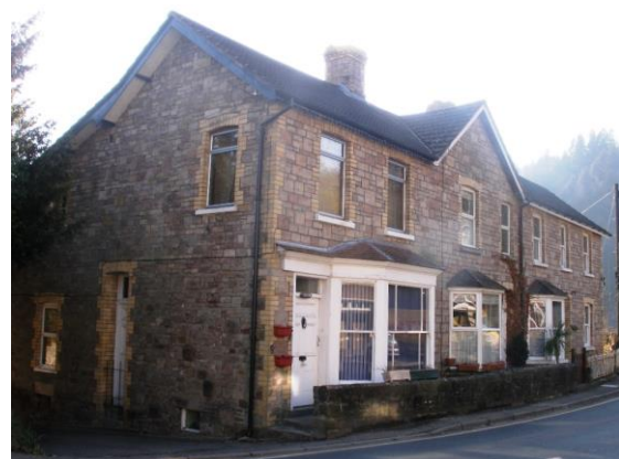
Fig.65 The terrace opposite the Wye Valley Hotel retains three cant bay windows. Buff brick dressings enliven the stone elevations.
