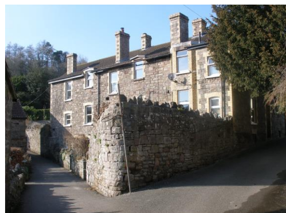
Fig.66 The rear of the terrace in Fig 16 reveals that it utilises the abrupt change in level with its basement storey. The Cat Brook is channelled under the building on the left hand side.
