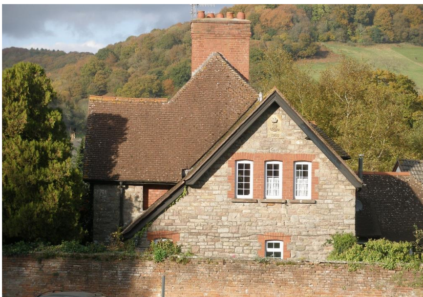
Fig.70 A Crown cottage built in 1903. This semi-detached Vernacular Revival inspired building uses well considered materials and creates a lively composition of hipped roofs and gables culminating in a sturdy brick chimney.
