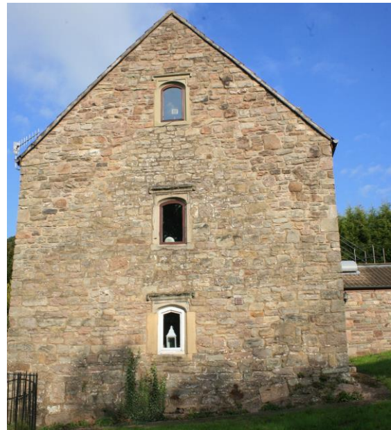
Fig.20 The distinctive local rubblestone with building alterations highlighted in varied pinker shade of stone
