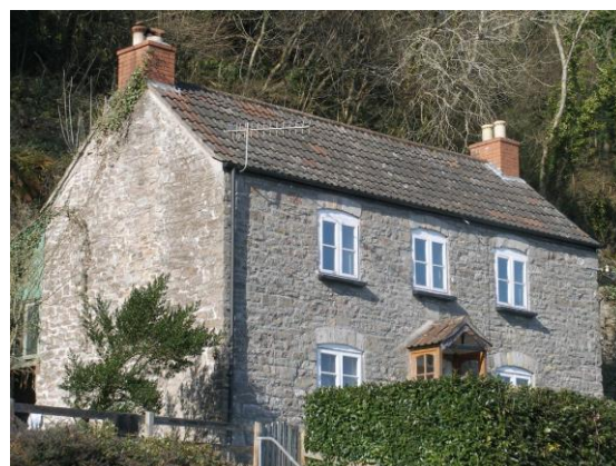
Fig.55 Cottage near the 'Moon and Sixpence' pub. Whilst many cottages have timber lintels, this has well formed 'soldier arches'
