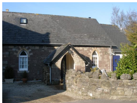
Fig.62 The former schoolhouse or hall adjoining the former chapel, also converted, but almost intact externally.
