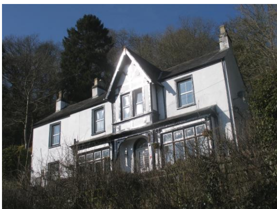
Fig.64 'The Old Rectory': a typical Victorian Gothic house with a gable and steep pitched roof. The rectangular projecting mullioned bays either side of the front door are an attractive feature.
