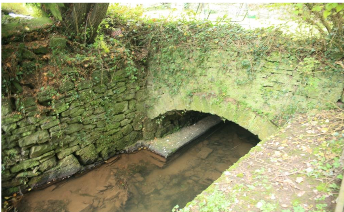
Fig.75 Stone lined stream culvert, one of many which wind their way down the Angiddy valley and through the heart of the former industrial core of Tintern
