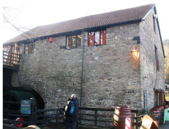
Fig.56 The Abby Mill. This substantial building fronts onto the main road at high level on the left. Note the waterwheel on the left.
