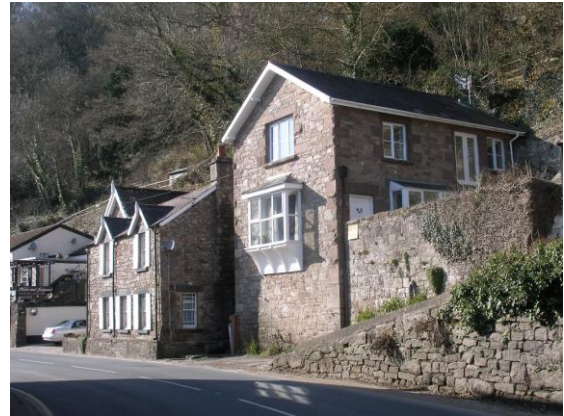
Fig.67 The Old Coach House, facing the river is well sited, creating a group with its neighbour and the large retaining wall. The well designed oriel window with its curved brackets is an eye catcher in the street scene
