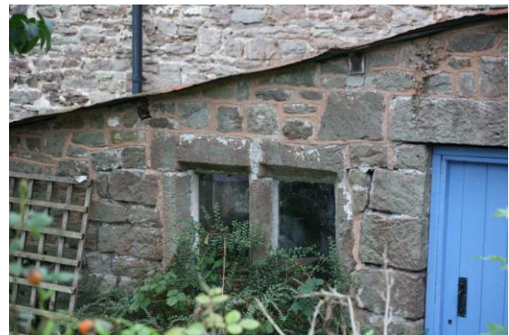
Fig.22 An historic stone mullion window in the lean-to attached to Fryers' Row
