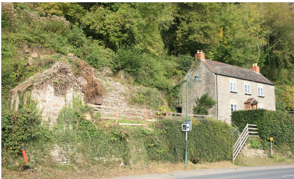
Fig.27 Spring Cottage set up above the road in a commanding position with stone outbuilding
